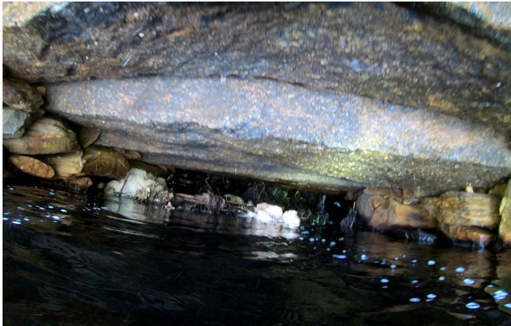
Photo 9 – Roof (Deck) Stones, Stone Abutments & Vegetation at Upstream (North) Opening
