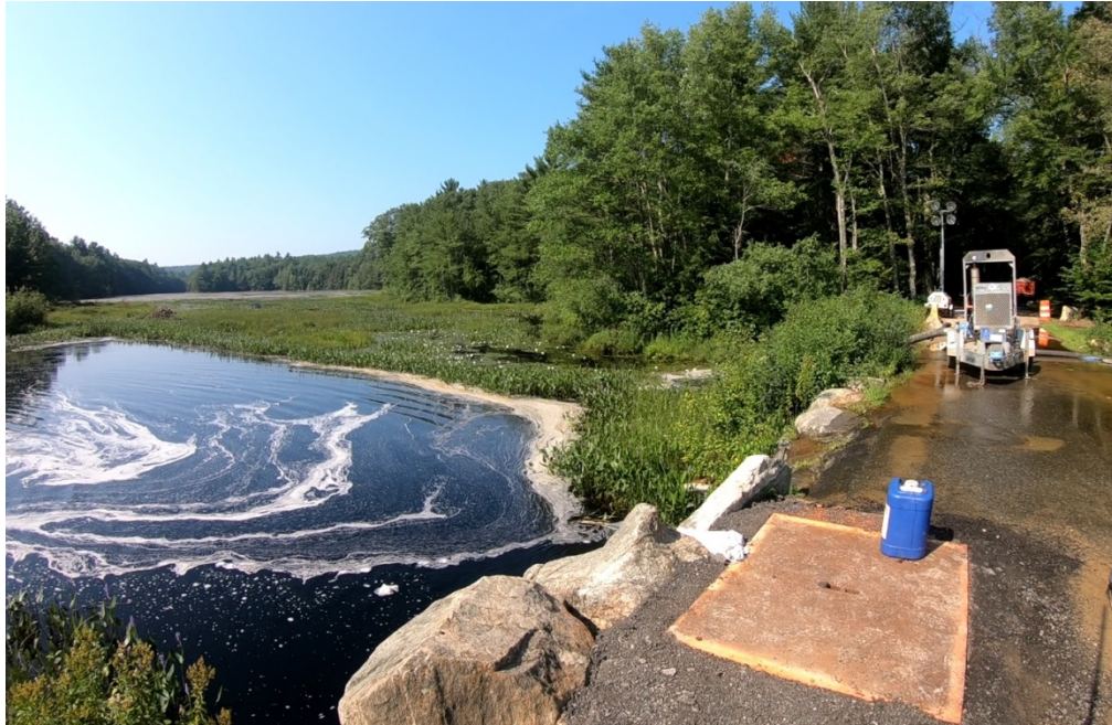
Photo 5 – Roadway Plate & Stream Overtopping Roadway
