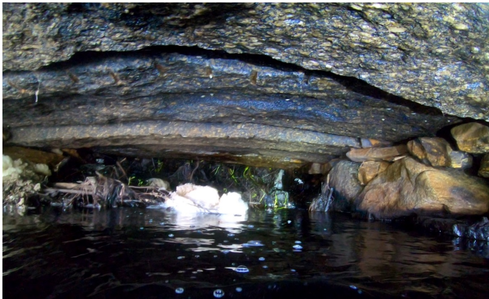
Photo 10 - Roof (Deck) Stones, East Abutment & Vegetation Blocking Upstream (North) Opening
