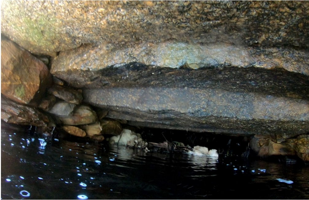
Photo 11 – Irregular Roof (Deck) Stones & West Abutment
