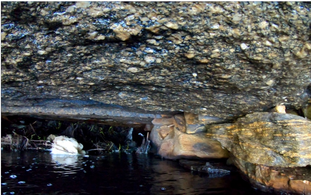
Photo 12 – Roof (Deck) Stones and East Abutment
