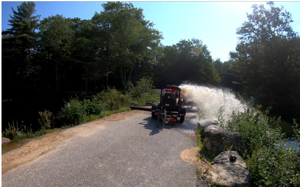
Photo 6 – One of Two 6" Diameter Pumps Discharging Downstream
