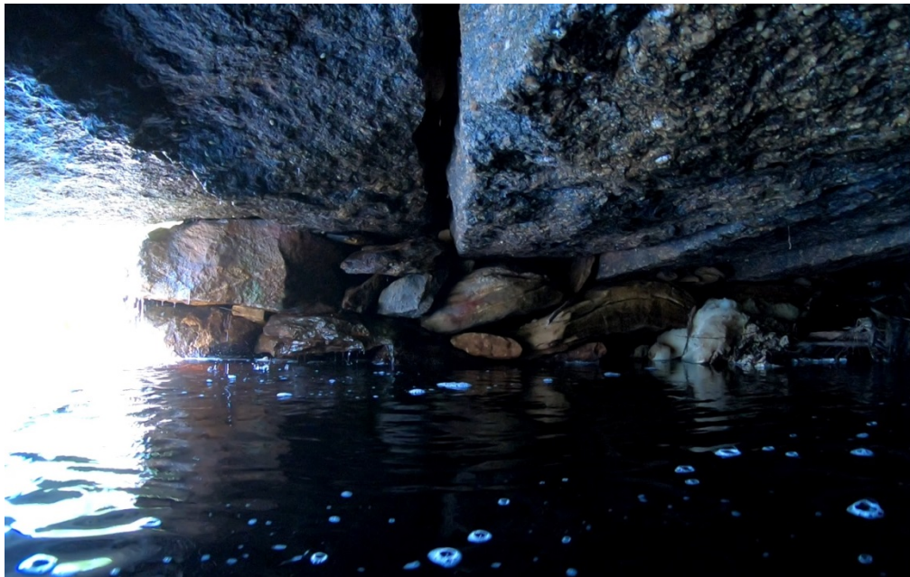
Photo 14 - Roof (Deck) Stones below Roadway Plate and West Abutment
