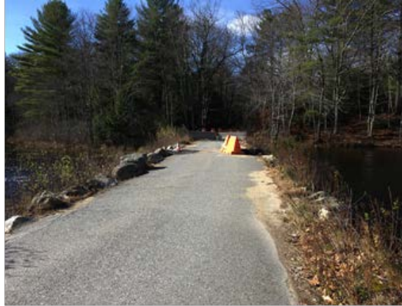
Figure 1: Looking west down Stoney Bridge Road over the existing culvert crossing
