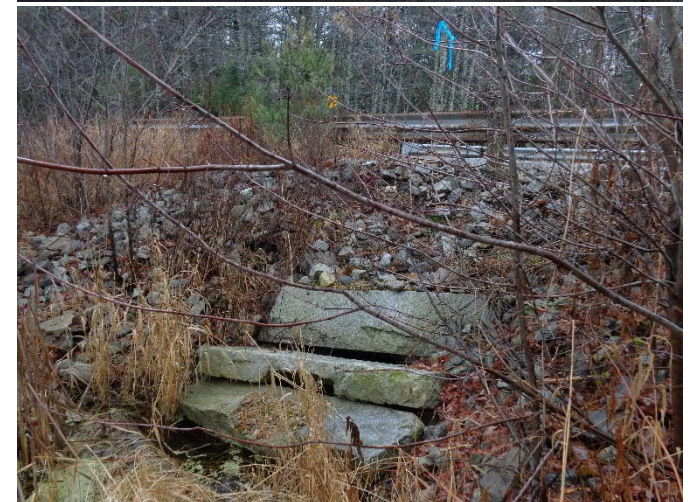
Collapsed headwall at a cross culvert
