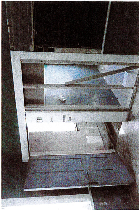
SOUTHEAST CORNER - LOOKING AT OPEN DOOR TO STAIR AND ATTIC ACCESS HATCH. OPPOSITE OF DOOR TO BE RESTORED WITH ABANDONED DOORWAY TO RIGHT TO BECOME CABLE RISER ACCESS WITH LOUVERED DOORS. WALL TO RIGHT TO HAVE CORK APPLIED BETWEEN WAINSCOT AND HORIZONTAL WOOD 1 X 6 TRIM TO BE INSTALLED AT DOOR HEAD LEVEL.
