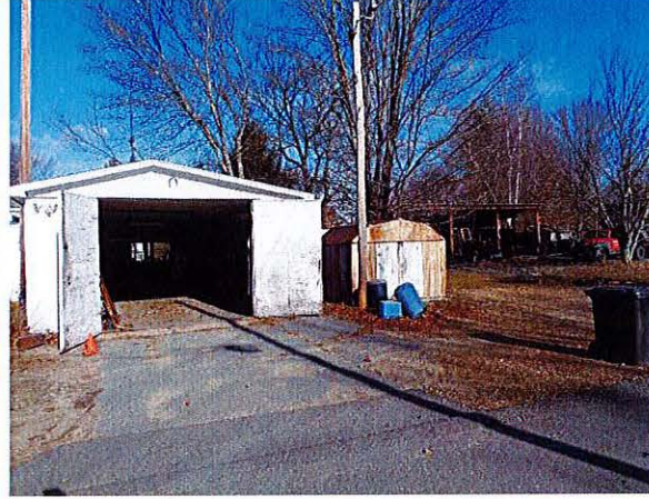
Garage at 711 Baldwinville, shed, and 0 Vernon St garage to far right.
