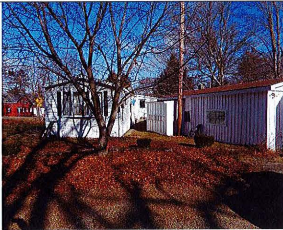
711 Baldwinville Mobile home on left, garage on right. Faces Vernon St.
