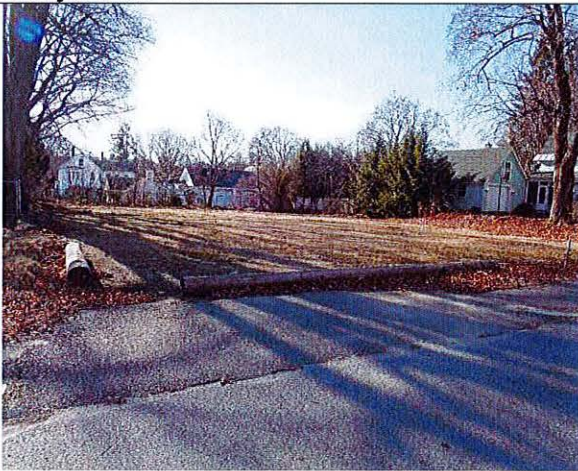
Subject curb cut for driveway – overgrown with grass.
