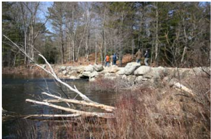
The Stone Bridge at Stone Bridge Pond
