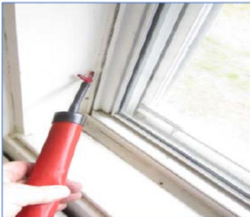
Left: Town Hall – testing of the windows indicates considerable air leakage at sashes. The metal-frame units need new weatherstrip installed. The older wood-framed units are not used, and therefore should be sealed shut, tightening these units, alleviating drafts, and improving occupant comfort and the building's overall energy performance.
