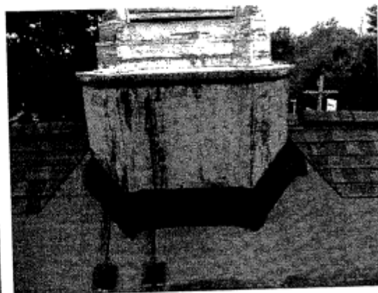
4. Base plinth from South – Galvanized steel sheetmetal painted to appear to be copper.
