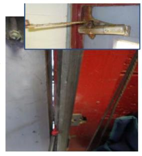
Right: Fire Sta. #1 – photo shows the deterioration of the sheetrock and wood eave framing at rear of the building. This is due to air and moisture leakage through the large openings in the upper walls (at the soffits/eaves, insert). These soffit openings need to be air-sealed and insulated to prevent air leakage through these openings and the subsequent condensation that
